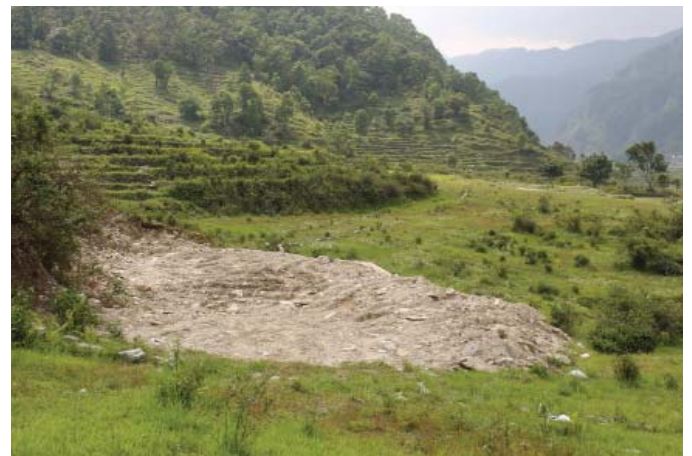
Photo (top): the Logged On team in Nepal, Bishow Adhikari, Chabbi Poudel and Ves Raj Bastola with Logged On's CEO handing over the money for the construction of the foundations of the new school; (bottom) the site of the new school in Suiket.
