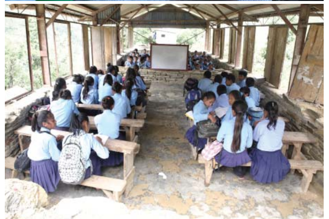
Photo (first two): water filter system installed at the Chhabdi school with the middle photo showing a training session for teachers and students on care and maintenance of the filters (thanks Kavita Thapa for the top photo); (bottom) walls removed from existing classrooms with truss frames and roof intact to make them safe for use at the Nabin school.
